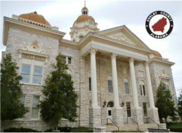
Shelby County Courthouse, Columbiana, Alabama.
